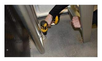
**Step 7**: Remove the assembled diving board and position the mount plates so the rivet nut is centered in the ½" holes.
